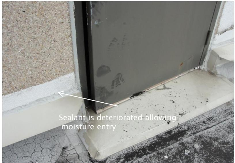
Sealant is deteriorated allowing
