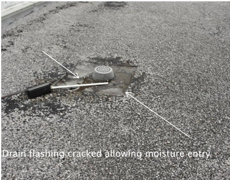
Drain flashing cracked allowing moisture entry
