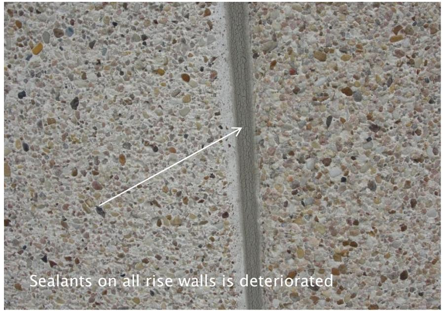
Sealants on all rise walls is deteriorated
